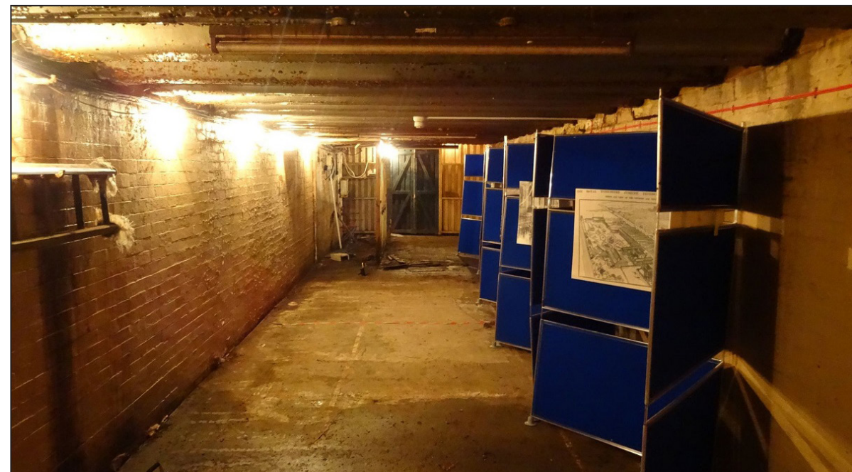
Saltaire tunnel- an important part of the World Heritage Site's history. Pic: Andrew C Bolt
