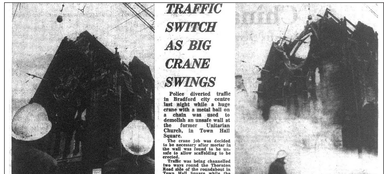
How the T&A reported the old building being brought down by a wrecking ball
