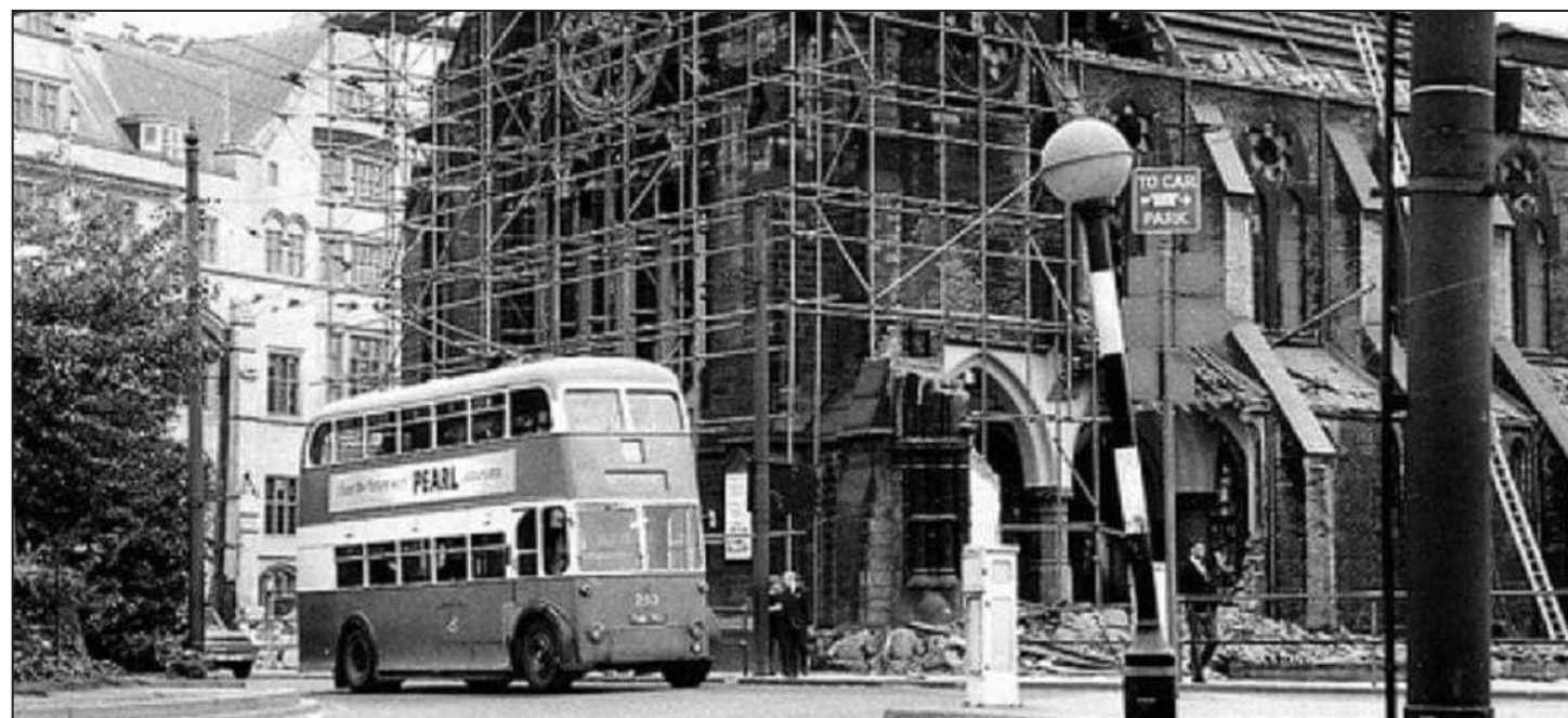
Scaffolding around the old Unitarian Chapel prior to its demolition
